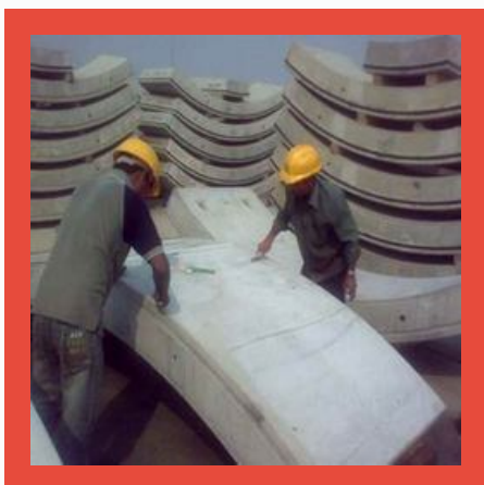
Protective Coating Services
