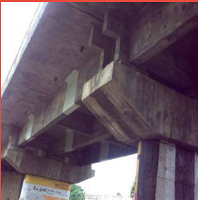
FRP Composites And Retrofitting
