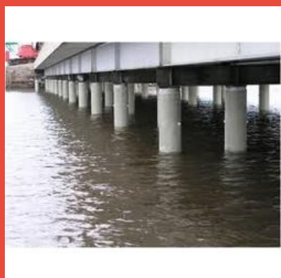
Advanced Pile Encapsulation
