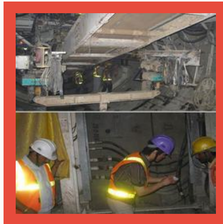
Underground Constructions And Tunneling Work
