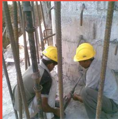
Anchoring And Groutings
