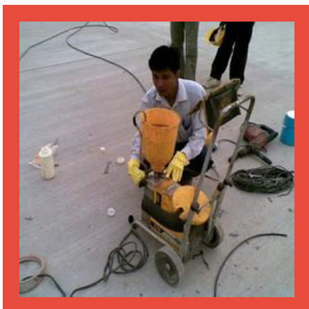
Injection Waterproofing Services
